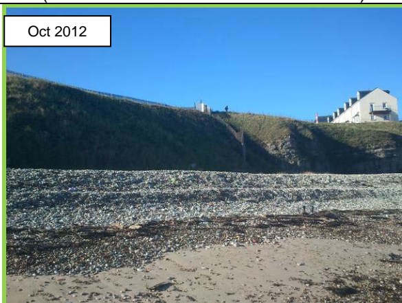
Undefended length south of beach ramp. (Asset Ref. No. 121AC901C0103C05)
