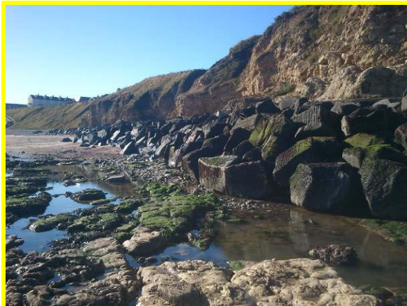
Rock armour protecting cliff toe tapers out (Asset Ref. No. 121AC901C0103C06)
