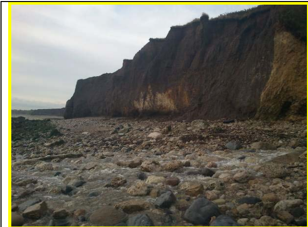
Looking south from Ryhope Dene. Frequent slumps and mudslides in upper till. (Asset ref. No. 121AB901B0804C01)
