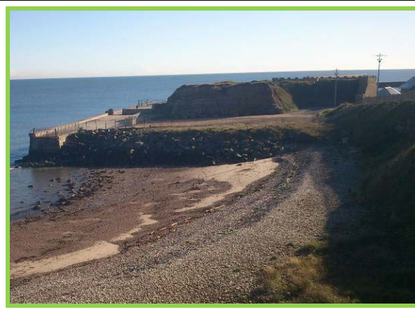
Rock armour at rear of harbour reclamation. (Asset Ref. No. 121AC901C0104C02)
