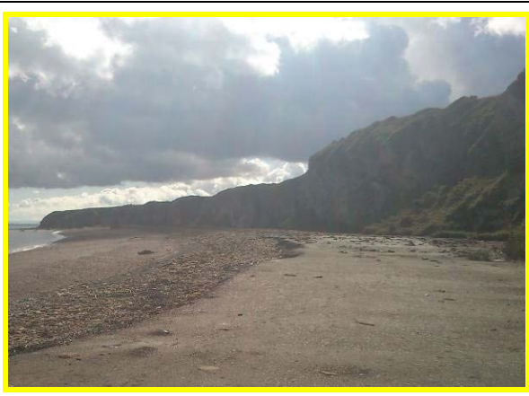
Blast beach looking south to Chourdon Point (Asset Ref. No. 121AC901C0107C01)
