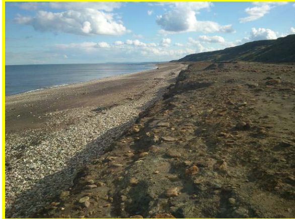
Eroding edge of colliery spoil at Horden Beach (Asset Ref. No. 121AC901C0201C02)
