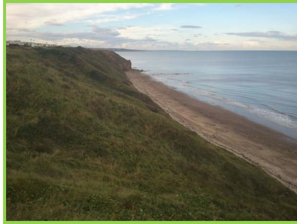
Vegetated cliff slopes adjacent to caravan park (Asset Ref. No. 121AC901C0301C01)
