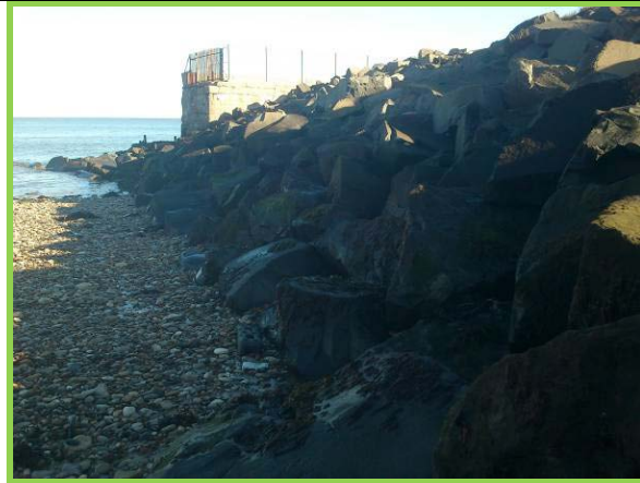
Rock armour in good condition (Asset Ref. No. 121AC901C0104C02)
