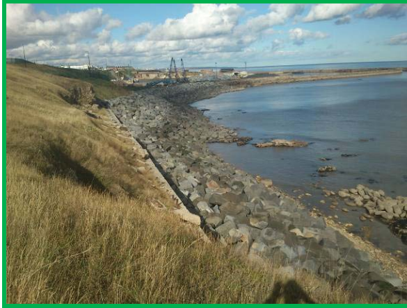
Rock armour south of port (Asset Ref. No. 121AC901C0105C01)
