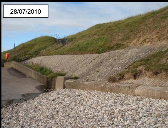
Wall at north end of Seaham. Photo from 2010 report.
