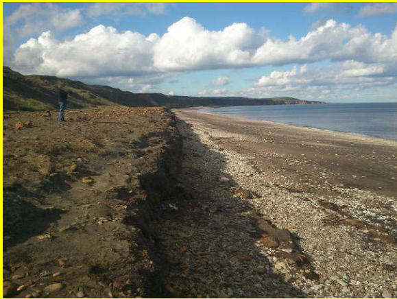
Eroding edge of colliery spoil at Horden Beach (Asset Ref. No. 121AC901C0201C02)
