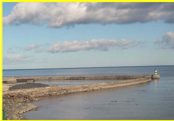
View of South Pier (Asset Ref. No. 121AC901C0104C17)
