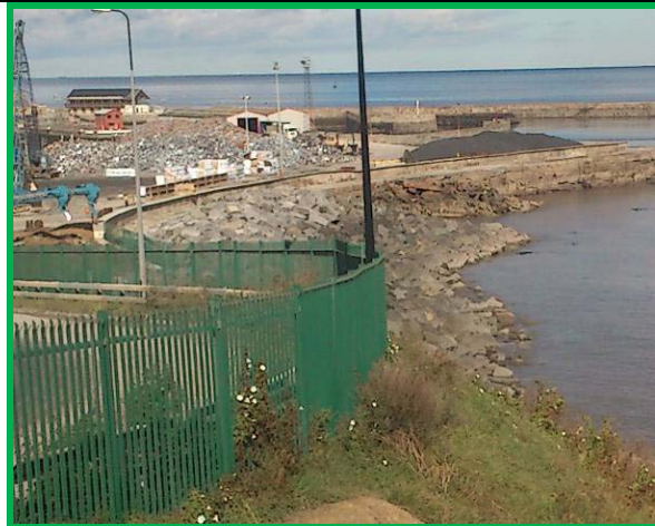
Rock armour at root of South Pier. (Asset Ref. No. 121AC901C0104C01)
