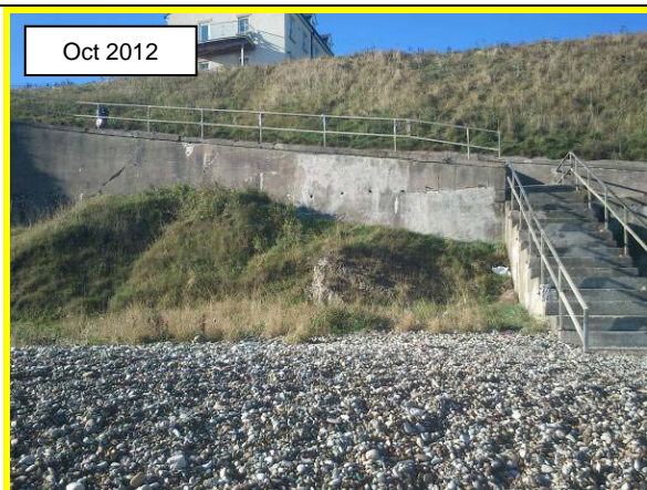
Beach access ramp and steps. (Asset Ref. No. 121AC901C0103C07)
