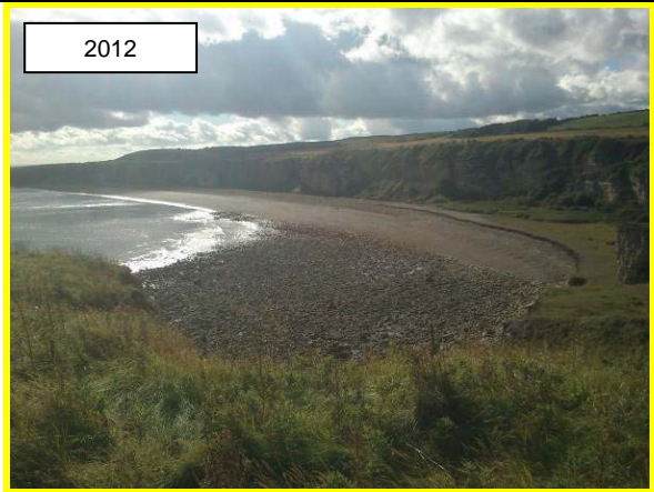
Eroding colliery Spoil at Blast beach (Asset Ref. No. 121AC901C0107C01)
