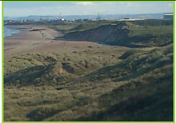
Sand dunes at Crimdon Beck, showing erosion of dune face to south (Asset Ref. No. 121AC901C0301C01)
