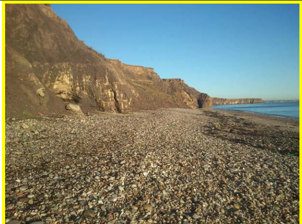
Looking north from near access steps. Mudslides covering sections of the limestone base. (Asset ref. No. 121AB901B0804C01)
