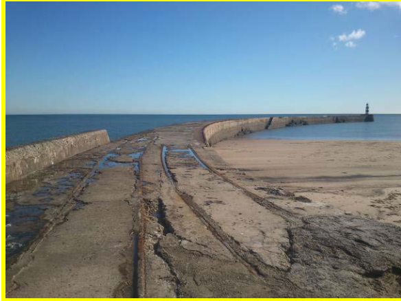
View of North Pier (Asset Ref. No. 121AC901C0104C03)
