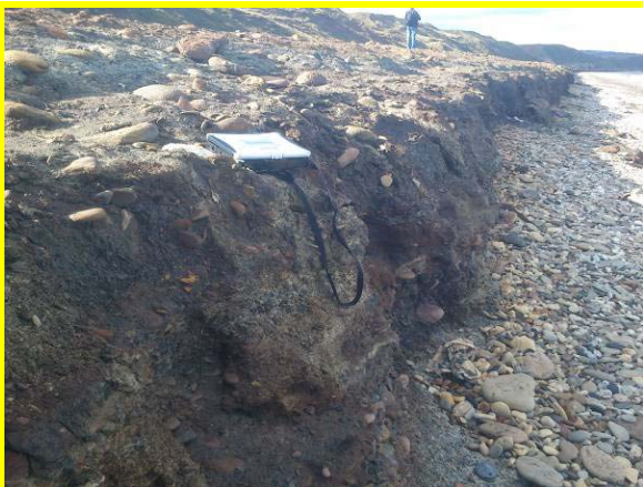
Eroding edge of colliery spoil at Horden Beach (Asset Ref. No. 121AC901C0201C02)
